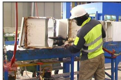
Fig. 5.48 Step 4: Removal of compressor
