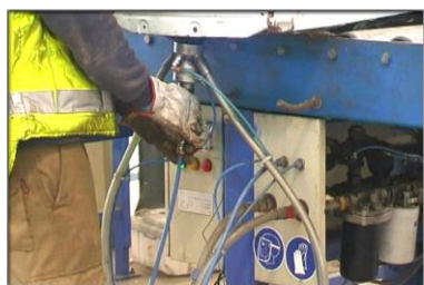
Fig. 5.47 Step 2: Removal of refrigerants and oil
